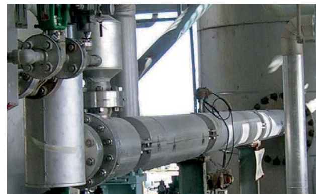
Fig. 1: Casale's AN2000™ pipe reactor
