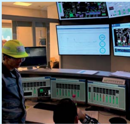
Fig. 5: Output from the soft sensor is displayed as a dashboard in the Engis plant's control room
