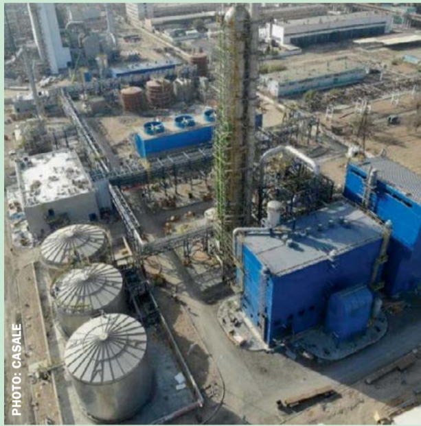
New JSC Navoiyazot nitric acid plant, Uzbekistan.
