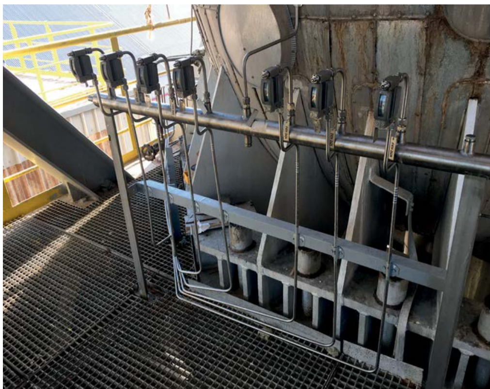
Fig. 2: Pressurised-type leak detection system. Header located at the bottom of a urea reactor. Flowmeters and control valves shown.
