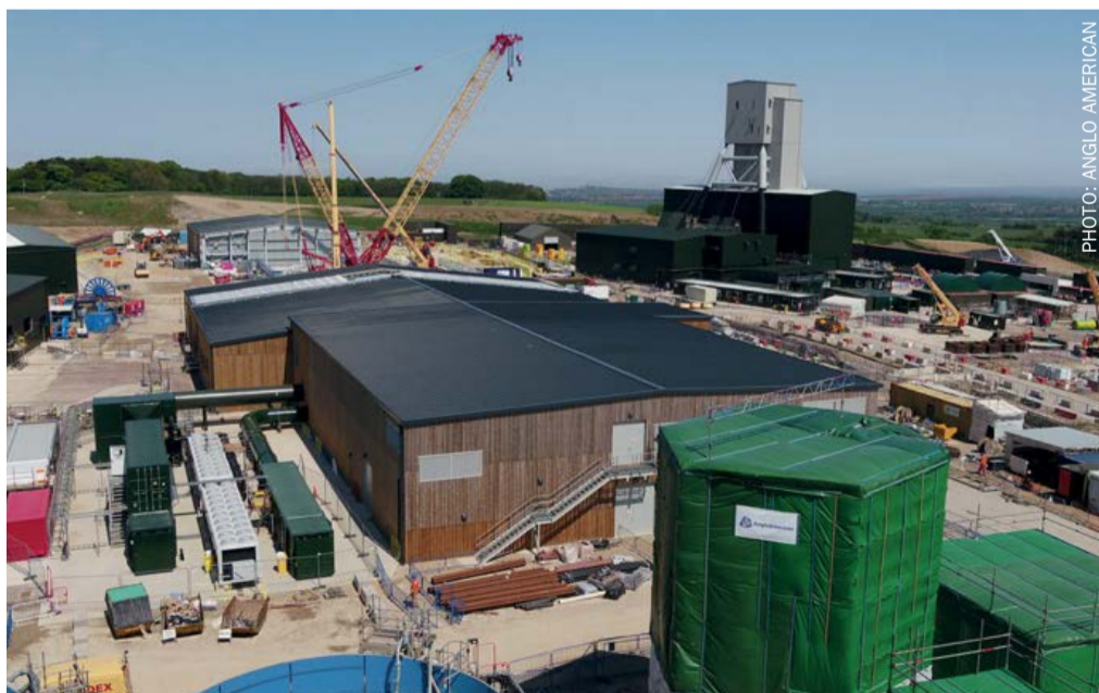
The under-construction Woodsmith polyhalite mine in the UK.
