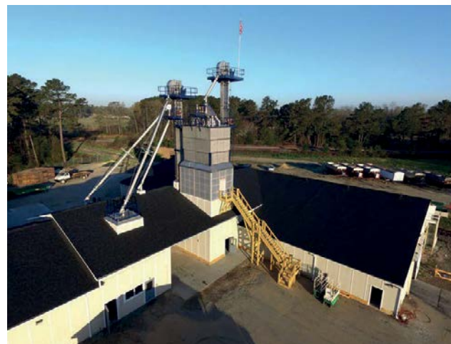
Sackett-Waconia tower blending system for FCI, North Carolina.
