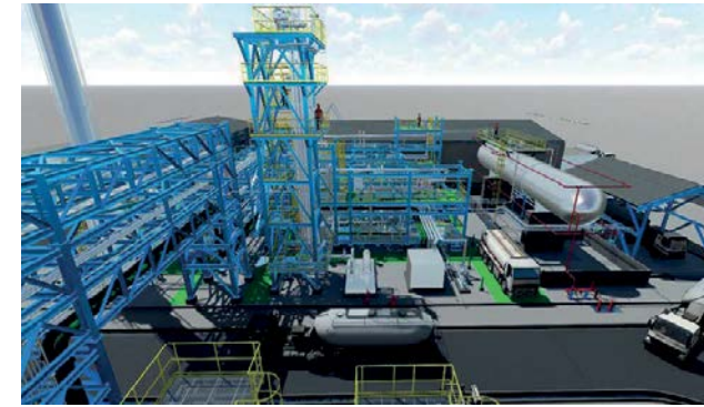
Fig. 1: Example of a thyssenkrupp Uhde small-scale modular green ammonia plant showing ammonia synthesis (centre) and pressurised ammonia storage tank (right).
