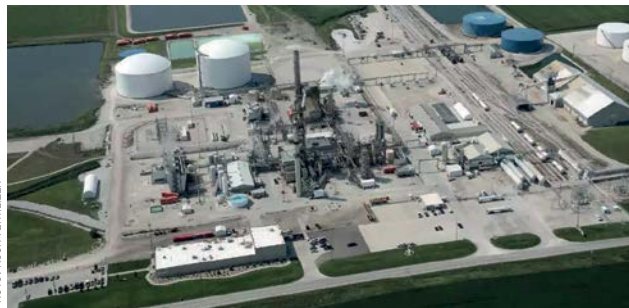
Koch Fertilizer recently commissioned a two-million-gallon ammonium thiosulfate (ATS) terminal at its Fort Dodge site in Iowa to support growing demand for liquid fertilizers.
