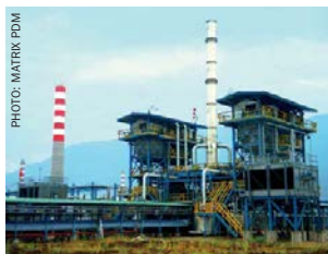
Above: Two Devco II wet prilling units, central China. These 8,600 t/d capacity units have a space-efficient, modular design.
