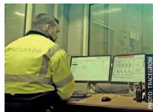
Control room of Tracegrow's battery recycling and fertilizer manufacturing plant in Finland.
