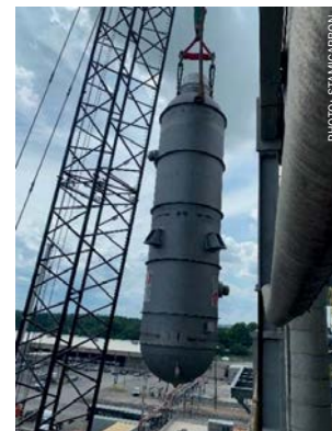
Fig. 3: Installation of a high-pressure after-reactor.
