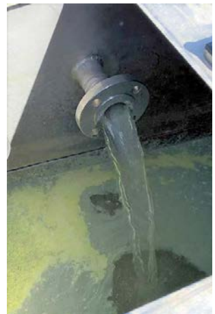
The waste discharge from the wet scrubbing system is recycled to the upstream sulphur seed generation system.
