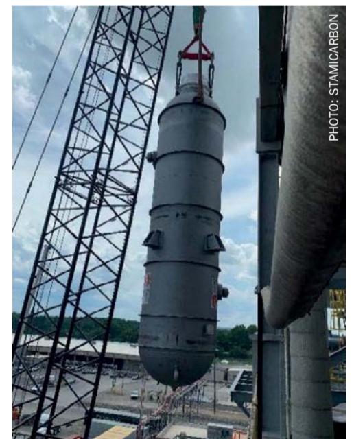
Fig. 3: Installation of a high-pressure after-reactor.
