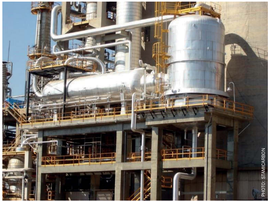
Fig. 2: Pool condenser in an Add-On structure that increases capacity.
