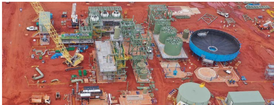
Construction at the Beyondie SOP project in Pilbara, Western Australia, early 2021.
