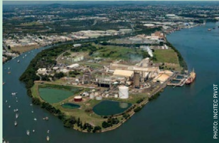
Incitec Pivot's Gibson Island plant, Queensland, Australia.
