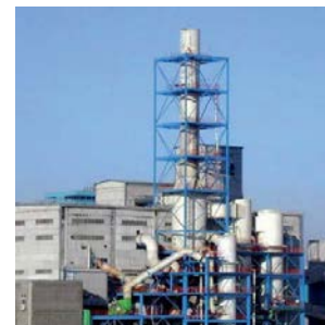
Casale dual pipe reactor granulation plant.
