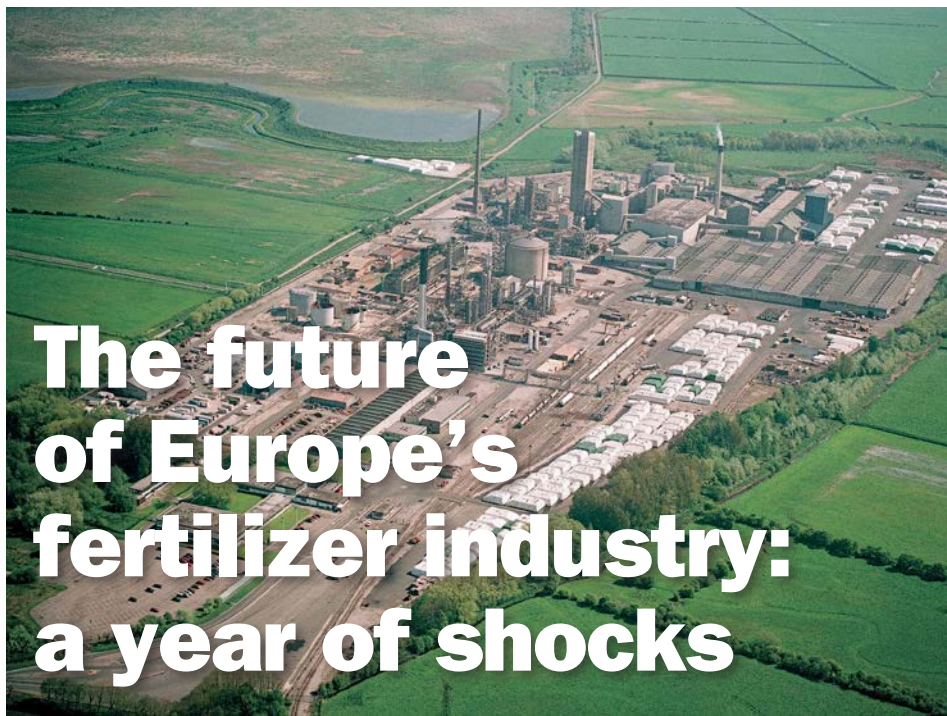
CF Fertilisers UK announced the closure of its Ince, Cheshire fertilizer production complex last June due to cost pressures.
