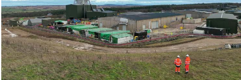
The under-construction Woodsmith polyhalite mine in the UK.
