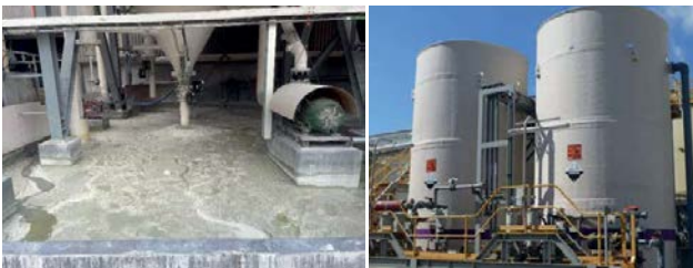
Silica-laden hydrofluorosilicic acid (FSA) (left) can be difficult to manage and even more difficult to dispose of. Armatec can help plant operators develop a zero effluent system (right) that provides FSA for re-sale for water fluoridation and/or recycling to the process.
