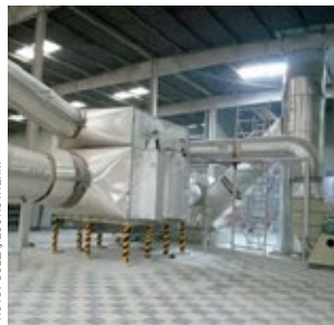
Photo: SOLEX/ECONOTHERM Econotherm's heat pipe heat exchangers can supply combustion air pre-heaters with recovered heat that is otherwise lost.
