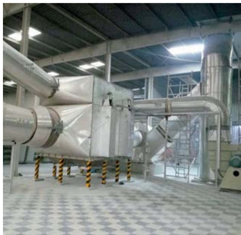
Econotherm's heat pipe heat exchangers can supply combustion air pre-heaters with recovered heat that is otherwise lost.
