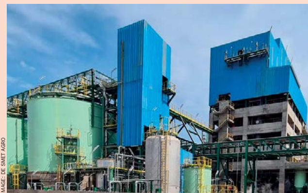
The Emaphos 2 purified phosphoric acid plant, Jorf Lasfar, Morocco.
