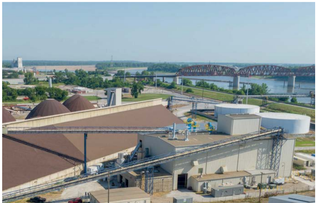
Ostara Nutrient Technologies recovers phosphorus from wastewaters globally to produce the struvite fertilizer Cystal Green.
