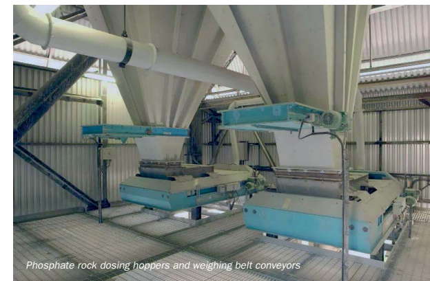
Fig 2: Overview of phosphate rock storage, handling & dosing
