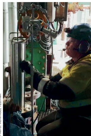
Fig. 1: Reformer pipe scanner operator.
