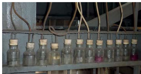
Fig. 1: A typical passive leak detection system.
