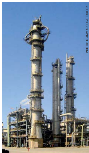
GV low-energy CO 2 removal unit.
