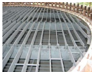
Fig. 10: Medium loading plant with no space for a pelleted secondary N 2 O abatement catalyst.
