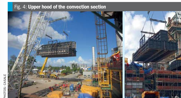
Fig. 4: Upper hood of the convection section
