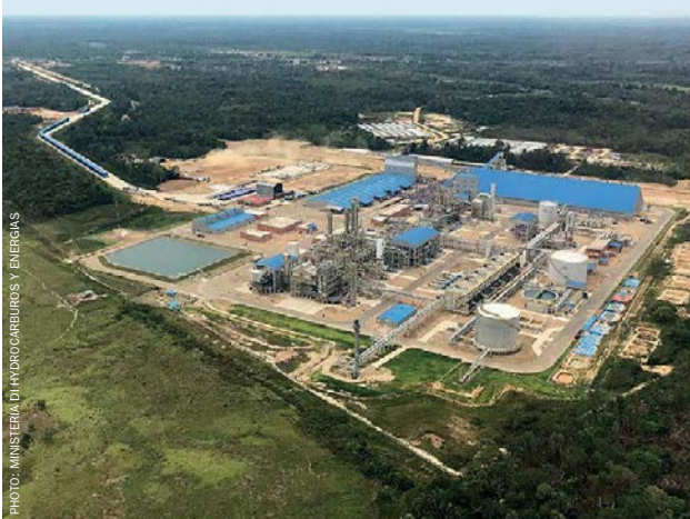
YPFB's urea plant at Bulu Bulu, Bolivia.
