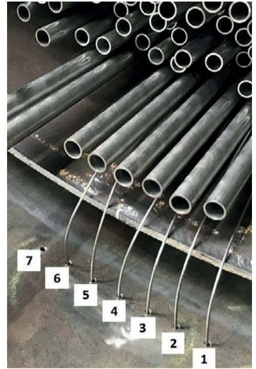
Fig. 5: Integration of ultrasound sensors into the CO 2 stripper.
