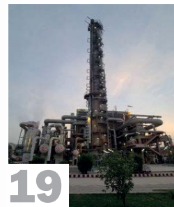
19 Nitric acid catalysts Monitoring to achieve optimum performance
