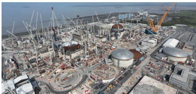
Construction of the new nuclear power plant at Hinckley Point C, UK.
