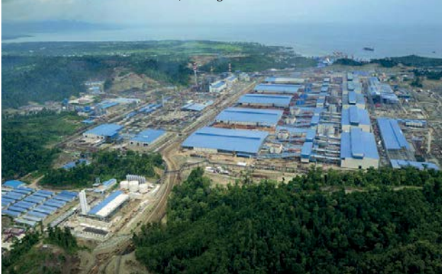
Indonesia's Morowali Industrial Park, showing HPAL units under construction.
