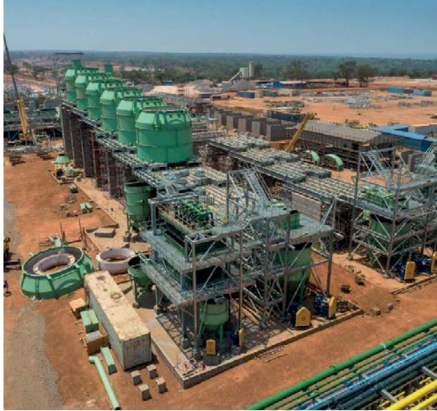
The Kamoa copper facility.
