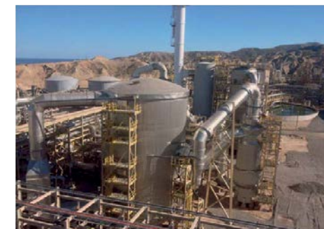
A sulphuric acid plant with HRS in a hydrometallurgical complex.
