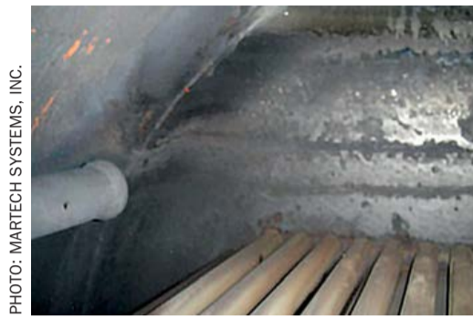
Fig. 6: Blowdown collection lateral
