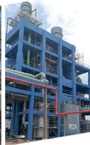
Phosphoric Acid Concentration Unit, Commissioned Oct 2021
