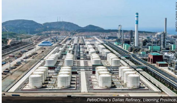
PetroChina's Dalian Refinery, Liaoning Province.
