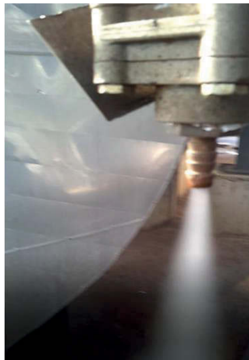
Fig. 8: White colour in the IAT outlet gas indicating \text{SO}_3 slippage.
