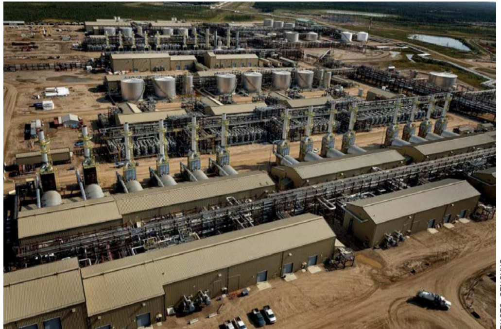
Oil sands processing at Cenovus' Christina Lake facility.
