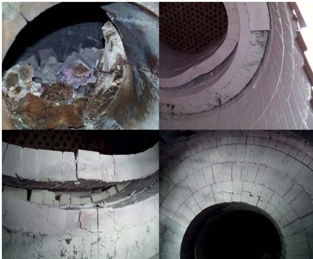
Fig. 7: Thermal reactor damage from liquid hydrocarbon carryover.
