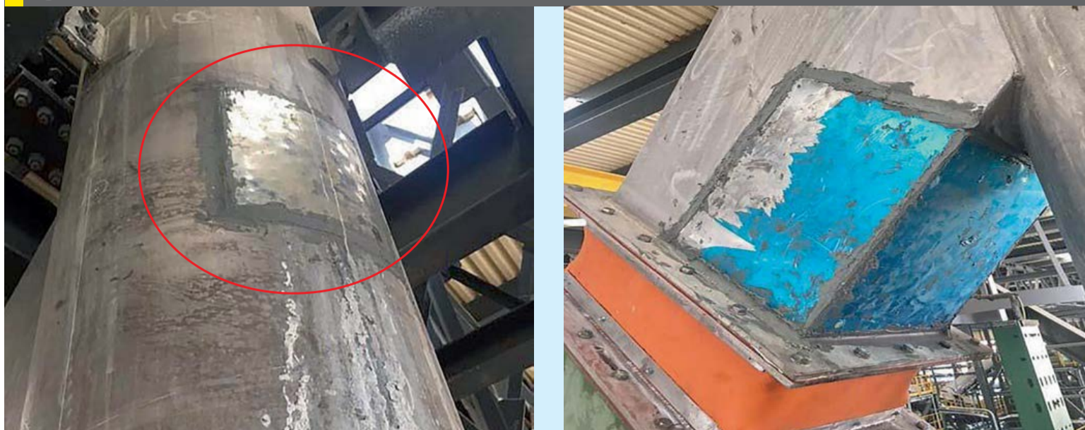
Fig. 3: Temporary repairs to scrubber outlet duct
