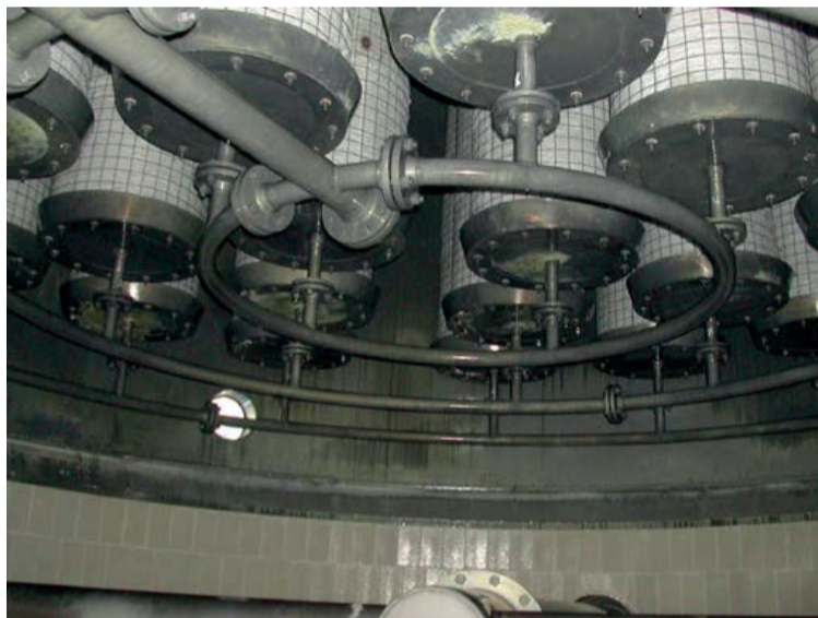
Fig. 7: Flanged type collection system with drip trays.
