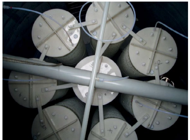
Fig. 8: WSA candle filters with wetting ring system.
