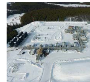
The Simonette gas plant, Alberta.
