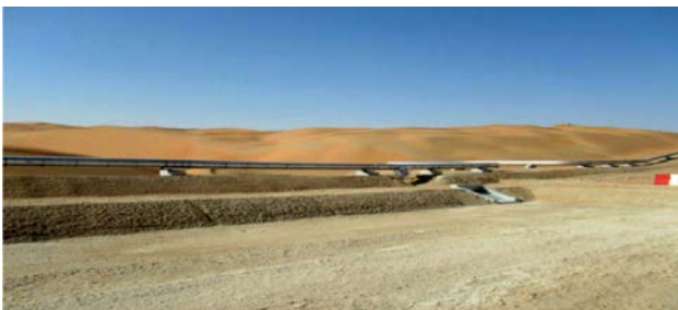
Fig. 7: Drain and drain pit for the new sulphur pipeline; 1 m elevation increase to avoid sand accumulation.
