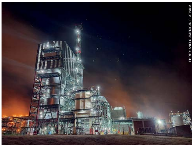
Fig. 3: The WSA unit at Anglo American's Polokwane smelter.
