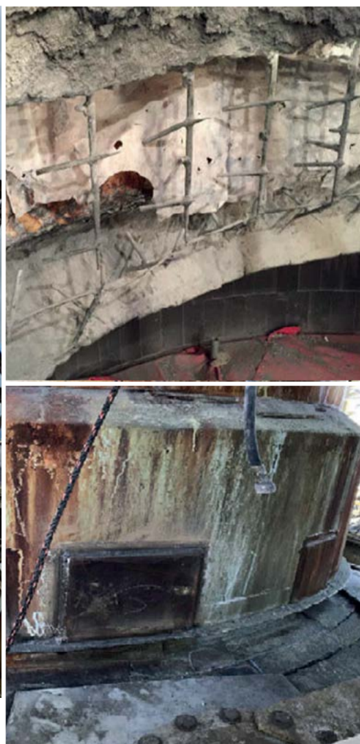
View of upper part of quench tower before replacement (above); damage to inside and outside of quench tower before replacement of upper part (right).
