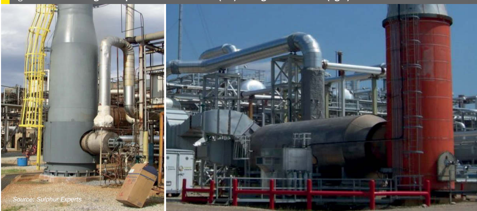
Fig. 6: Incinerator design examples – low 'K' incinerator (left) and high 'K' incinerator (right)
