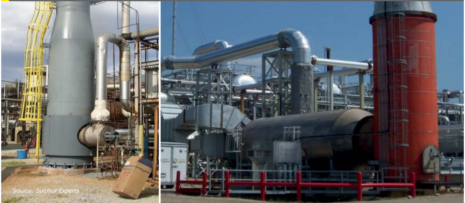
Fig. 6: Incinerator design examples – low ‘K’ incinerator (left) and high ‘K’ incinerator (right)
