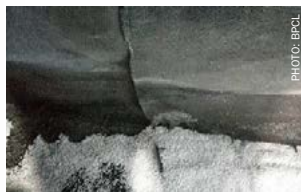
Fig. 5: Loose mesh near bottom grid
