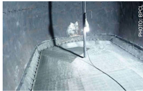
Fig. 9: Bottom grid after mesh modification
