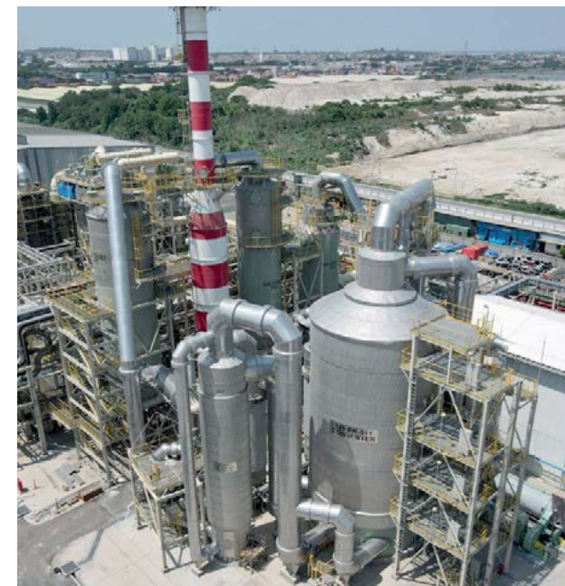
PT Smelting's acid plant expansion, Gresik, Indonesia
