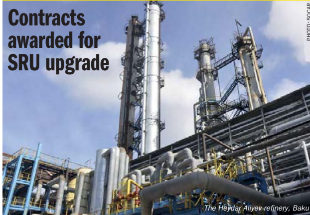
The Heydar Aliyev refinery, Baku
