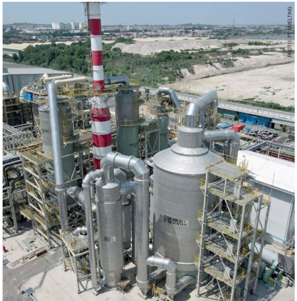
PT Smelting's acid plant expansion, Gresik, Indonesia
