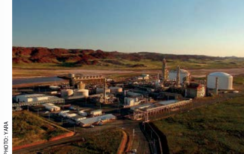
PHOTO: YARA Yara’s Pilbara ammonia plant, Western Australia.
