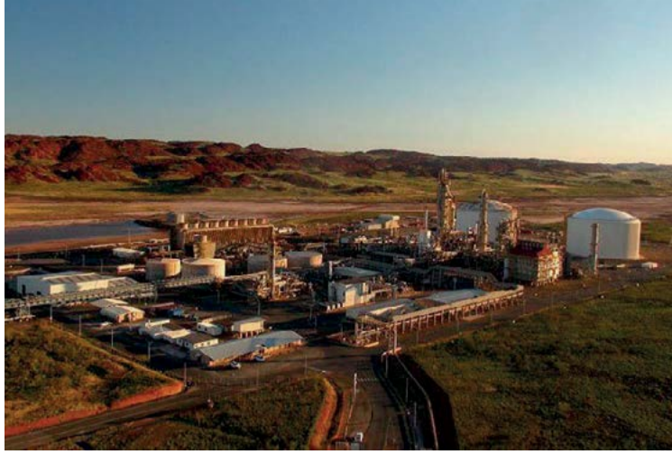
Yara's Pilbara ammonia plant, Western Australia.
