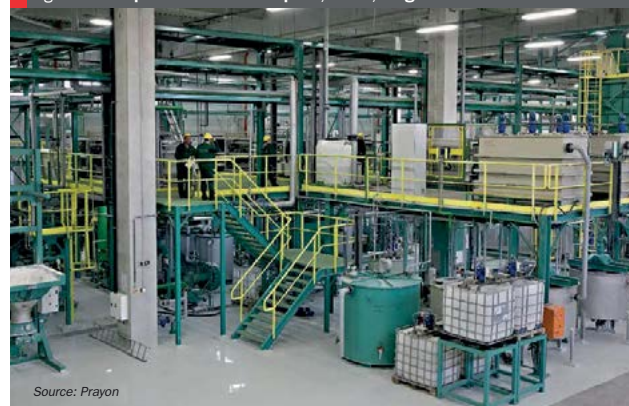
Fig. 6: Technophos semi-industrial plant, Varna, Bulgaria
