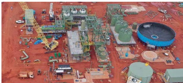
Construction at the Beyondie SOP project in Pilbara, Western Australia.
