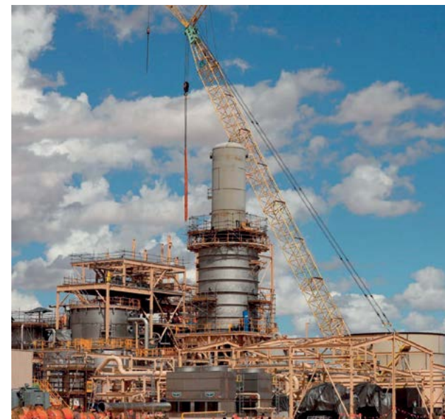
Erection and installation of a SOP crystallisation plant at Lake Way, Western Australia.
