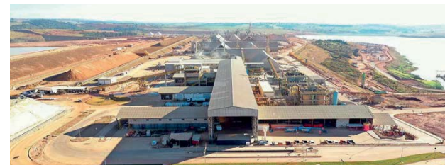
Yara's flagship Serra do Salitre phosphate project, Minas Gerais, Brazil.
