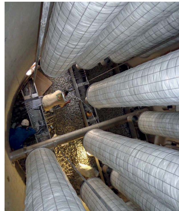
A view of the MECS® Brink® mist eliminators in the new acid tower.
