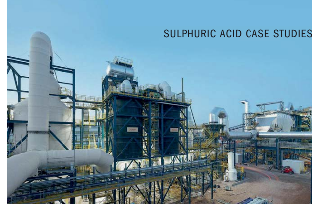
Mazidagi's gas cleaning plant section.
