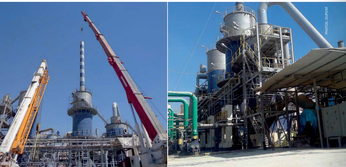
Left: The new tower as it is lifted into place at Unit 6. Right: Since start-up, Unit 6 has operated to performance guarantees, producing up to 640 t/d of acid.
