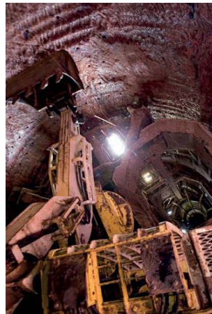
Galloway shaft sinking platform and potash layer, Esterhazy.
