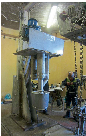
Fig. 1: First industrial VSB installation
