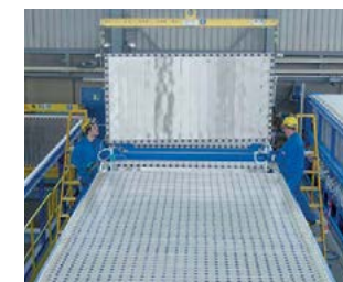
Electrolyser installation by Thyssenkrupp Steel.
