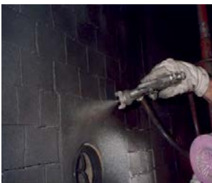
Fig. 14: Ceramic coating application on refractory brick lining.
