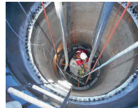
Fig. 4: Catalyst loading operator inside the cartridge during loading work.
