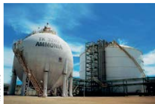
Left: Ammonia storage at NFC, India.
