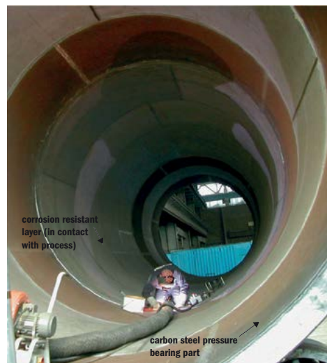
Fig. 1: Installation of a stainless steel loose liner in a urea reactor.
