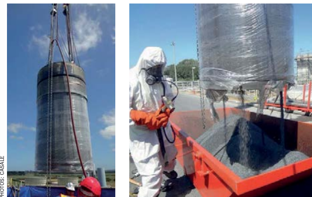
Above left: Fig. 6: Lifting of the basket full of active catalyst purged with nitrogen.
