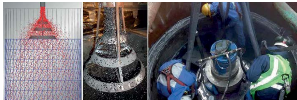
Fig. 5: Loading of tkIS uhde process ammonia converters.
