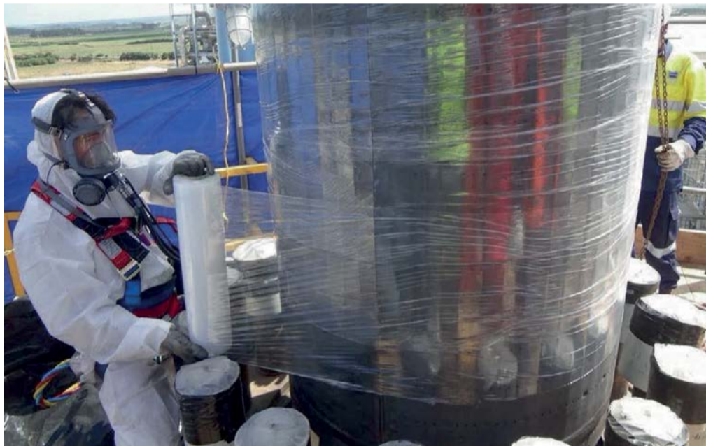
Fig. 5: Lifting of basket full of active catalyst purged with nitrogen – plastic wrapping to avoid the catalyst coming into contact with oxygen.
