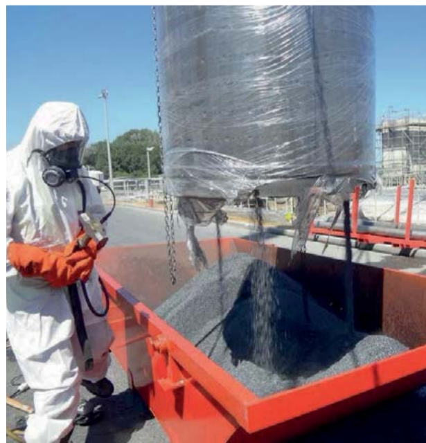
Above left: Fig. 6: Lifting of the basket full of active catalyst purged with nitrogen.
