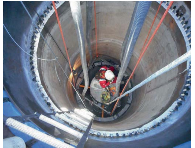
Fig. 4: Catalyst loading operator inside the cartridge during loading work.
