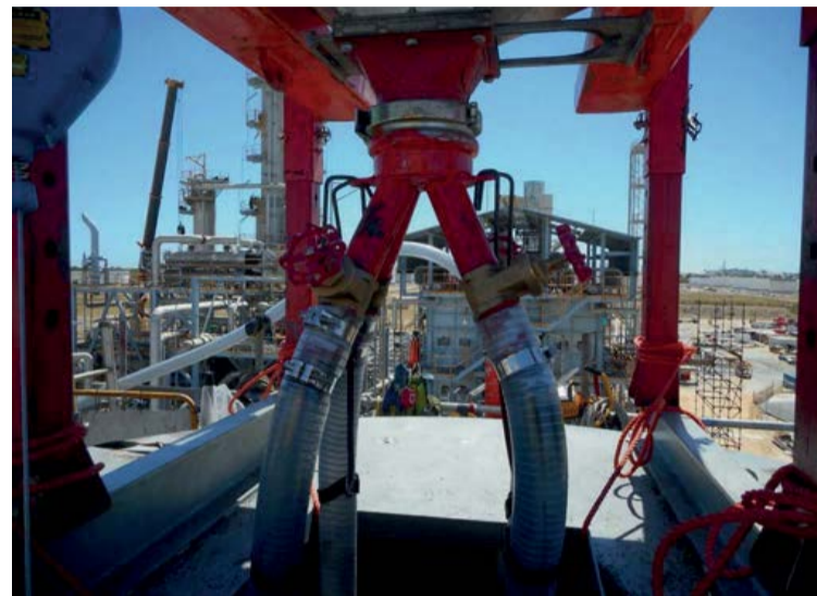
Above left: Fig. 1: Casale dense loading tool. Above right: Fig. 2: Detail of the fixed hopper on the converter top with details of valves for catalyst flow adjustment and hoses for catalyst feed.
