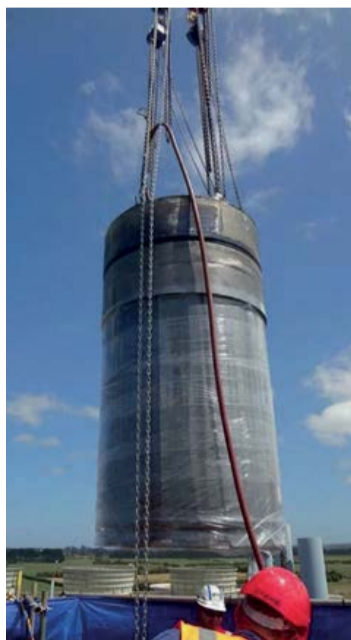
Above left: Fig. 6: Lifting of the basket full of active catalyst purged with nitrogen.
