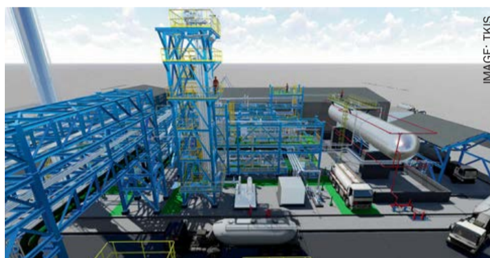
Module structure of a small-scale green ammonia plant from thyssenkrupp Industrial Solutions. Centre: ammonia synthesis; Right: pressurised ammonia storage tank.
