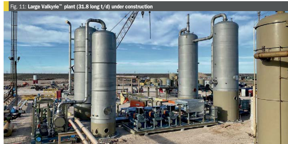
Fig. 11: Large Valkyrie™ plant (31.8 long t/d) under construction
