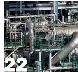
22 Ammonia processing Applications of SCO units in refineries and petrochemical plants.
