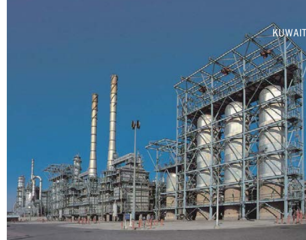
Mina Abdullah refinery.
