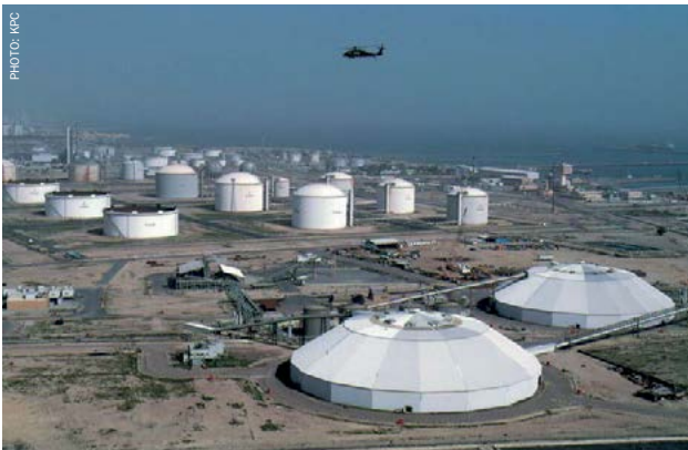
The tank farm at Mina Al-Ahmadi.
