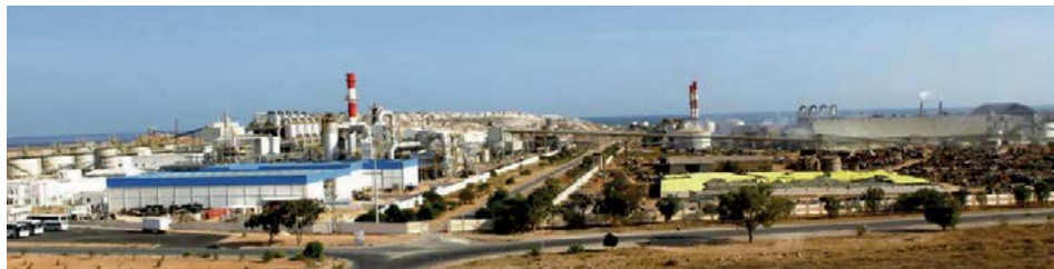
GCT's phosphate plant at Gafsa.
