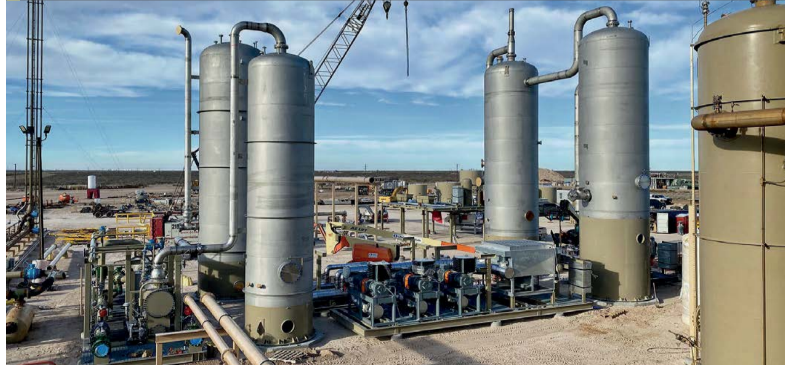
Fig. 11: Large Valkyrie™ plant (31.8 long t/d) under construction
