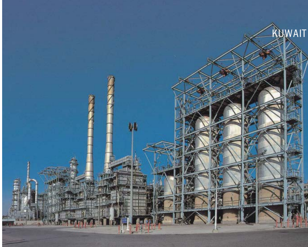
Mina Abdullah refinery.
