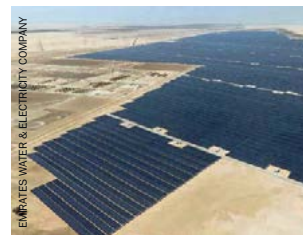
The Noor Abu Dhabi solar plant, largest of its kind in the world.
