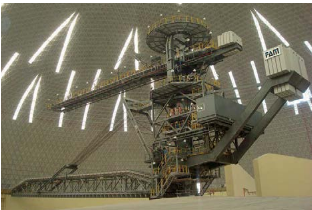
Left: The sulphur storage dome at Ruwais, with the stacker-reclaimer.
